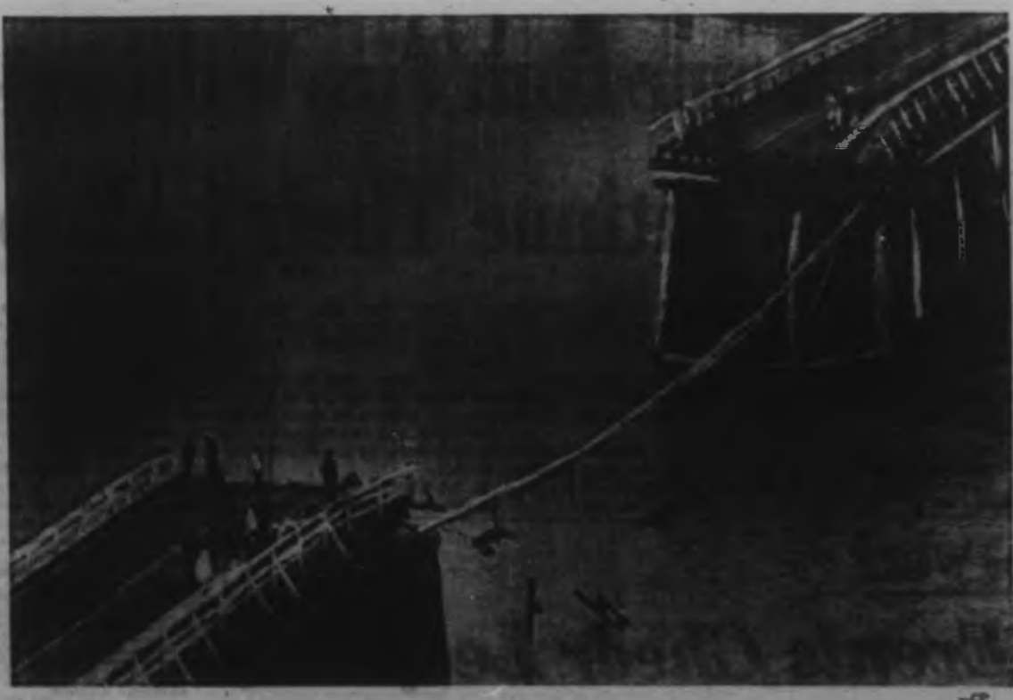
Muddy Fraser flows through gap in bridge
